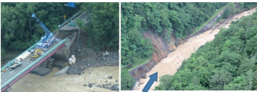
*Collapses of a bridge and a road by rapid flow created by heavy rainfall along the Chubetsu River in August 2010. Courtesy of Hokkaido Development Bureau.*
