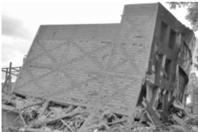
Tilt of building due to soft story formed in the first floor
