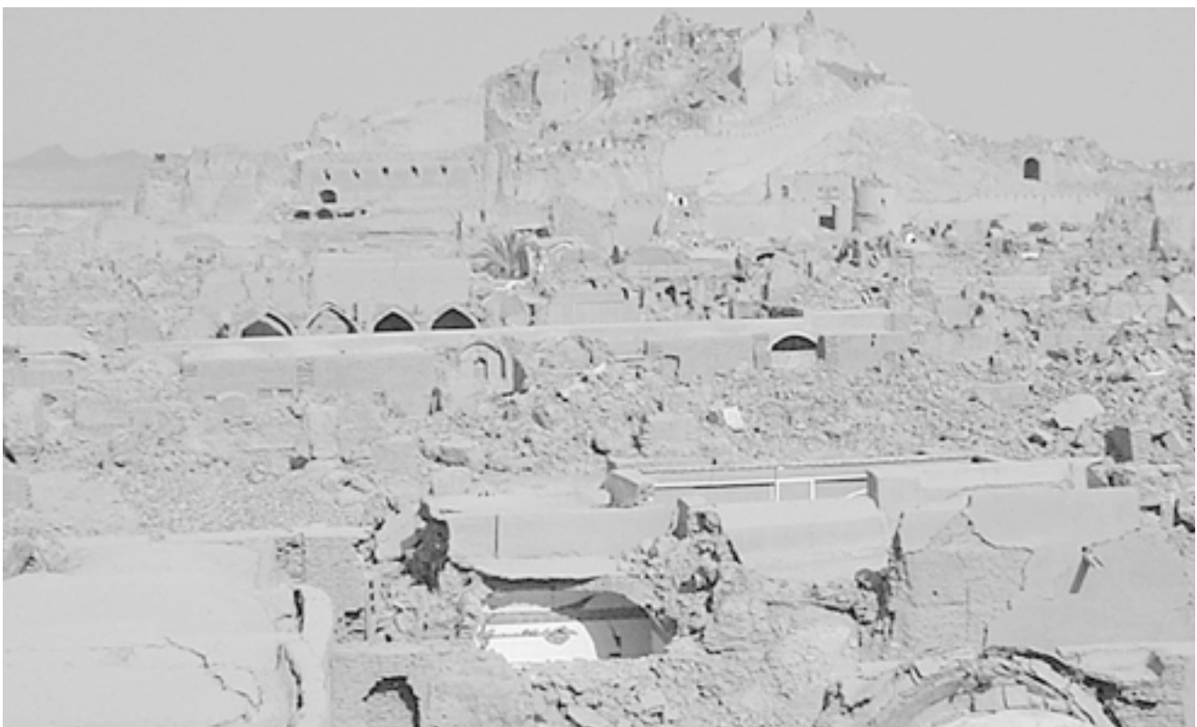
Earthquake-damaged view of historical adobe citadel (Arg-e-Bam)
