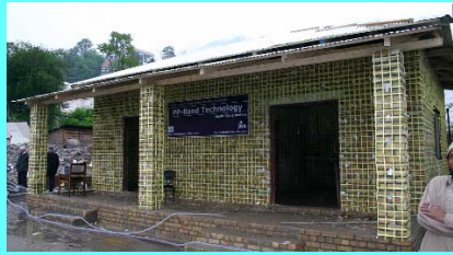
House model retrofitted with PP-band mesh in Kashmir area
