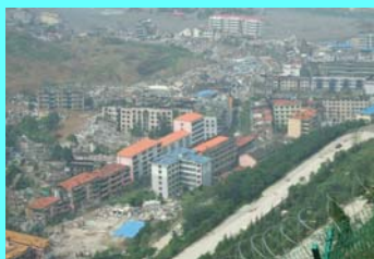
Devastating damage caused by the 2008 Sichuan Earthquake (Photo courtesy of Prof. K. Konagai)
