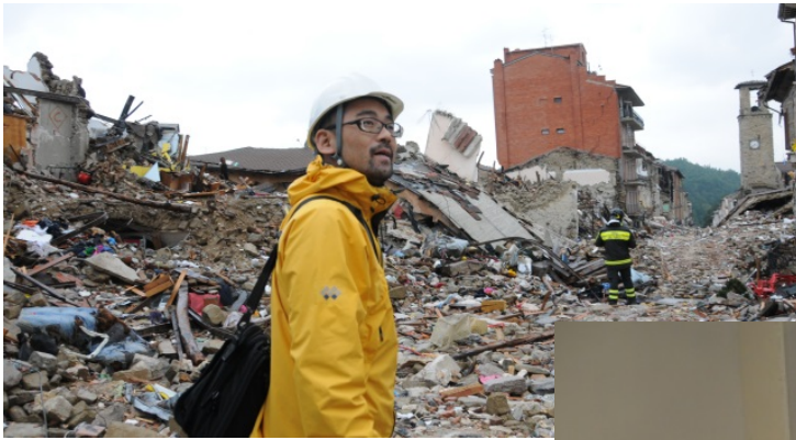
Photo 1: Damage survey in Amatrice
